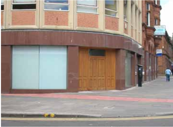
Inactive façade, John Finnie Street
