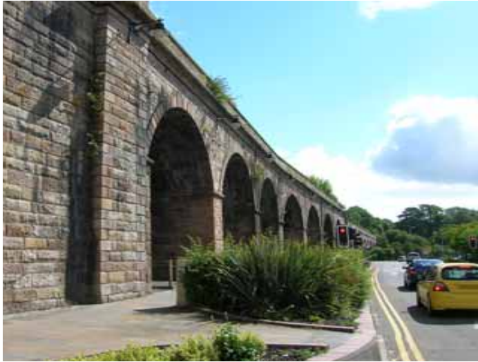
Kilmarnock Railway Viaduct
