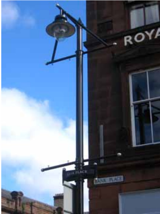
Street Lighting, Bank Place
