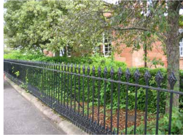
Cast iron railings at the Procurator Fiscal's Office
