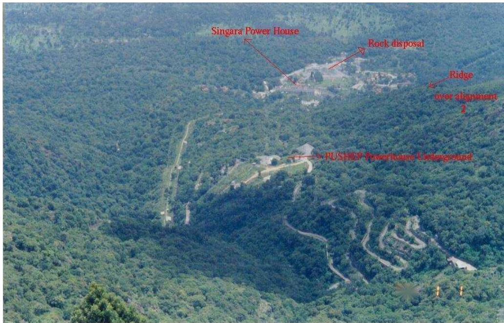
Figure 7.1: A View of PUSHEP location from Glenmorgan.
