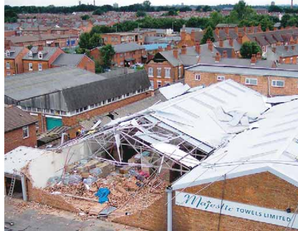
● The tornado ripped through the roof of Majestic Towels' premises on Alfred Street, Sparkbrook.
