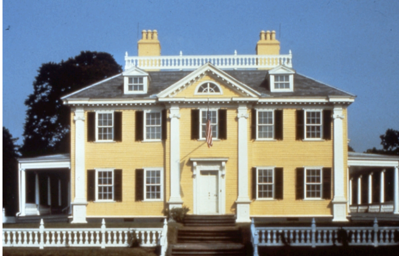
Courtesy of the National Park Service, Longfellow Historic Site
