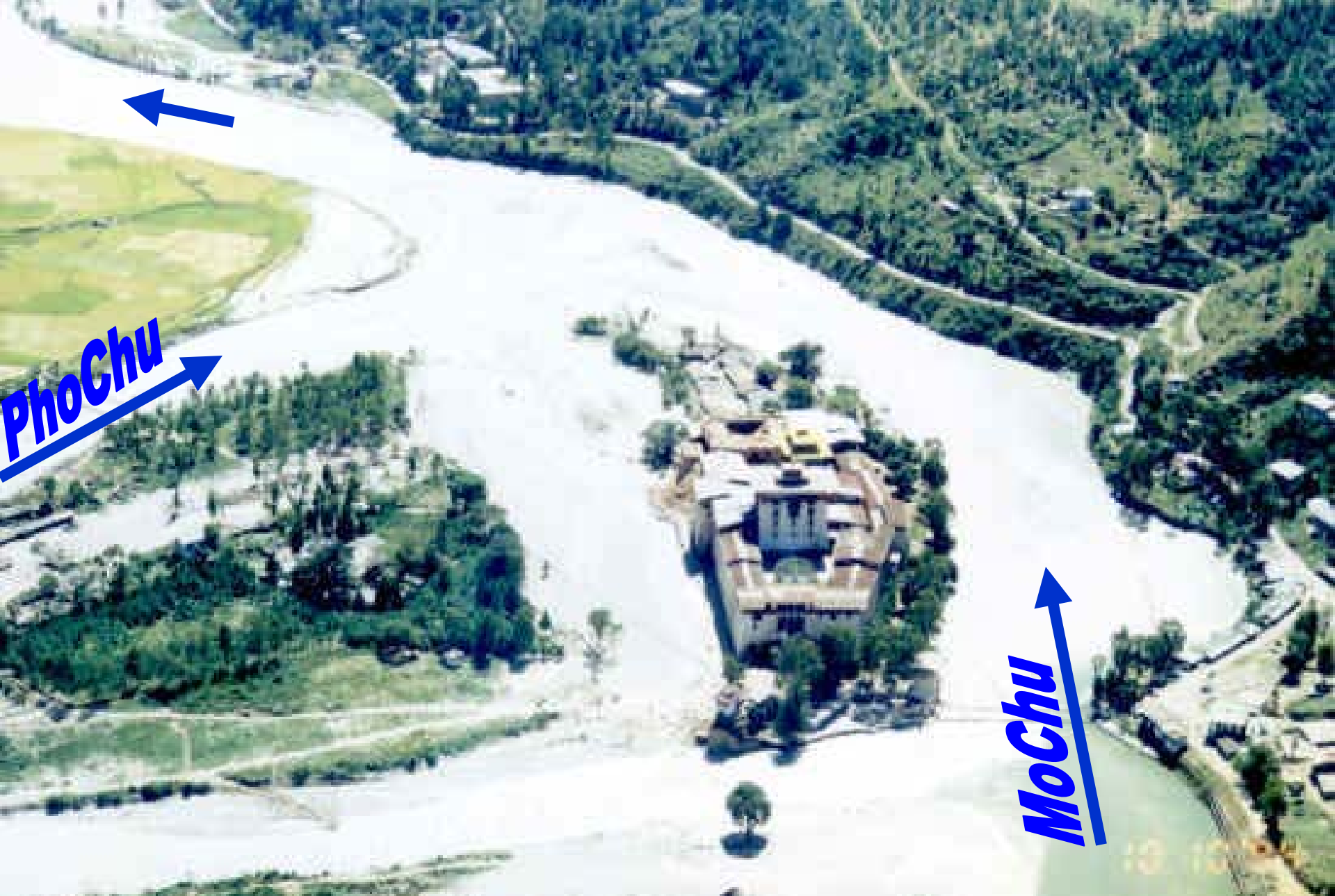
Punakha Dzong after 1994 GLOF from Luggi Tsho. It shows the confluence of Pho Chu and Mo Chu below the Dzong and the scars of the back flow water after it had joined Mo Chu and dammed the flow above the Dzong (Photo source: Mr. Phuntso Norbu, 1994 three days after the GLOF)
