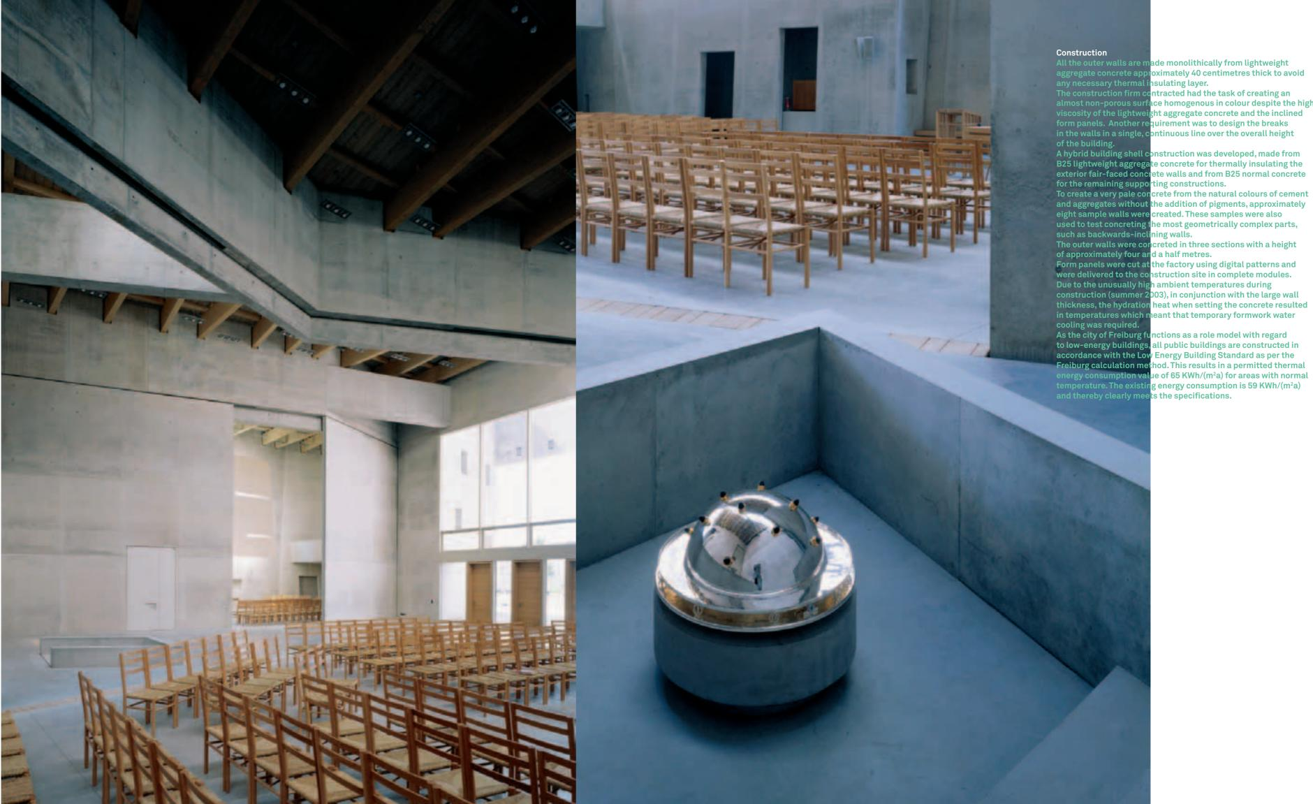
All the outer walls are made monolithically from lightweight aggregate concrete approximately 40 centimetres thick to avoid any necessary thermal insulating layer.
