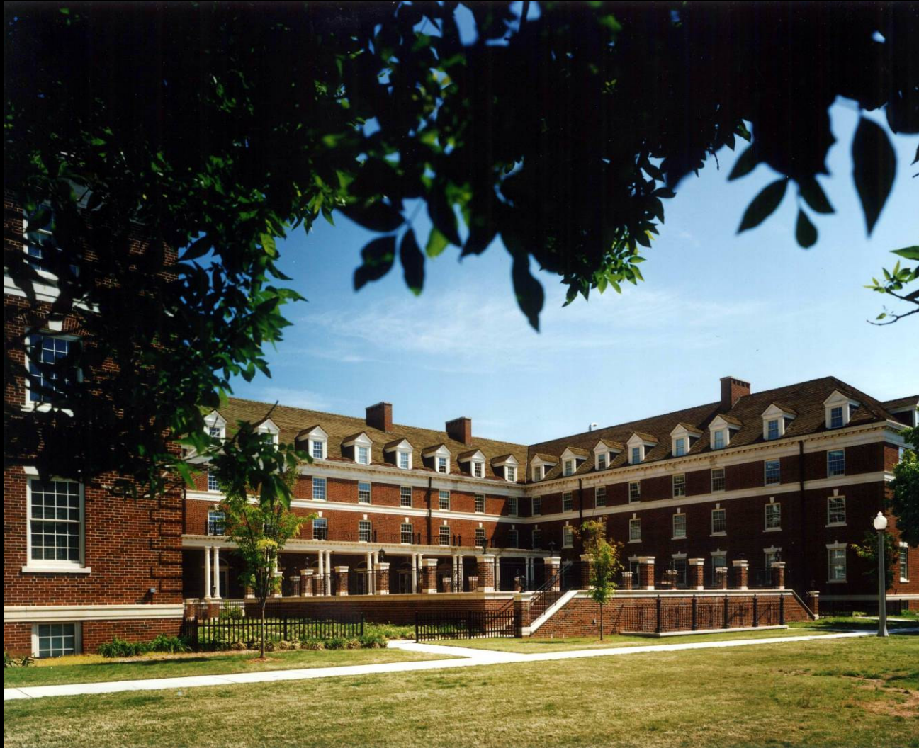
Willard Hall Renovation – view of south side
