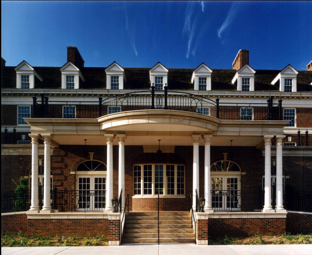
Willard Hall Renovation – new entry
