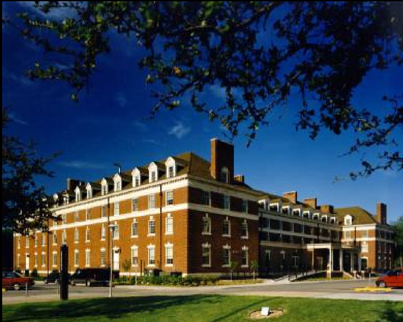
Willard Hall Renovation – view looking southwest
