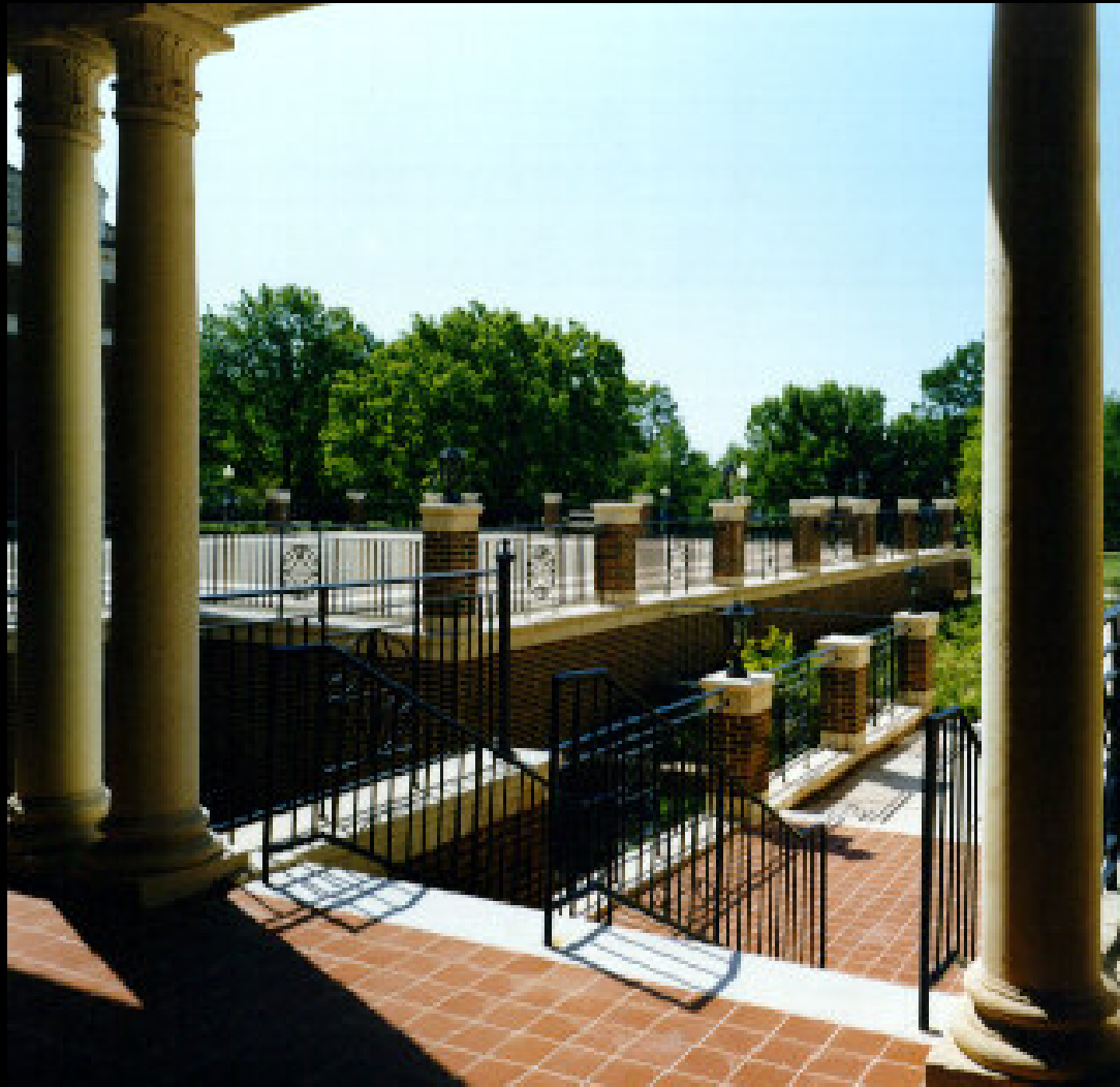
Willard Hall Renovation – new plaza
