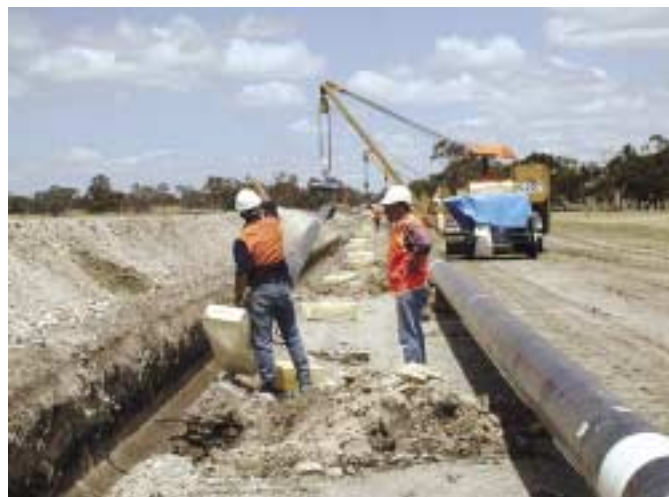
Laying of the SEA Gas pipeline near Tintinara. (Photo 49043)
