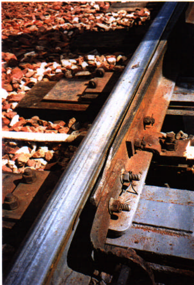
Figure 11: Carriage on points which are clearly set for loop.
