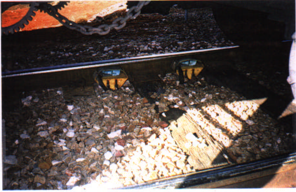
Figure 15: Proximity switches on main.
