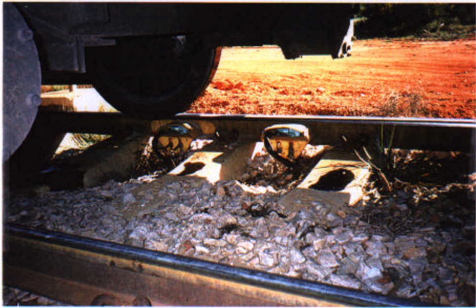
Figure 16: Proximity switches on loop.
