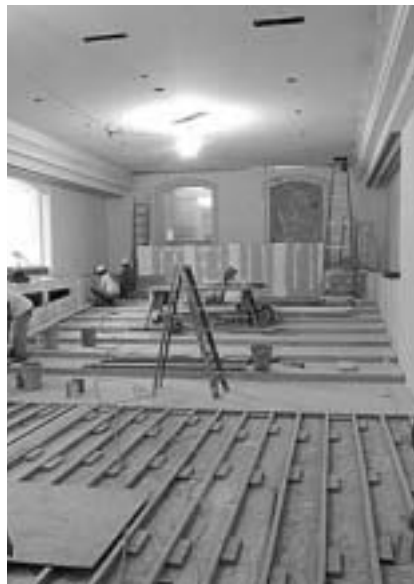
Drywall is installed in the Cohen Davison Theatre
