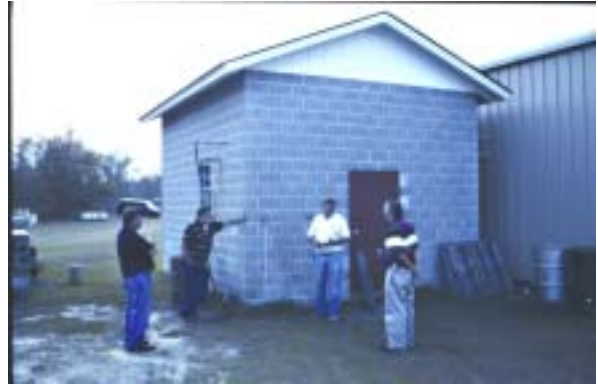
This concrete block building has been built to house a tank to store high fructose corn syrup. The operation utilises between 23-24 thousand lbs of syrup per year. Stored in warm conditions to prevent crystallisation. Reg Wilbank's honey house, Georgia.
