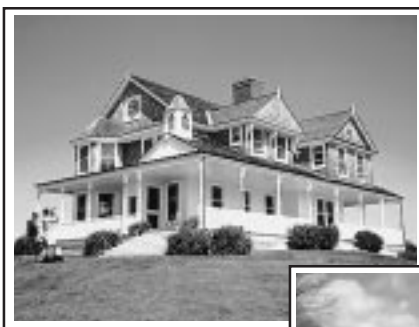
Tick Hall reconstructed - 2001
