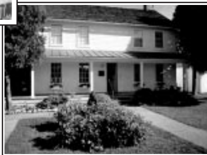
A state grant will help rehabilitate Harriet Tubman's home and the Home for the Aged (pictured above) in Auburn.
