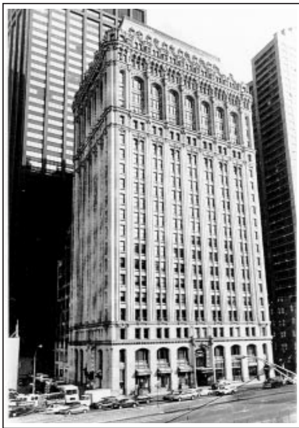
Located just south of the World Trade Center site, the West Street Building was among those severely damaged when the towers collapsed on September 11. Designed by prominent New York City architect Cass Gilbert and built between 1905 and 1907, this distinguished early 20 th century skyscraper is one of the fifty-one historic resources that the SHPO staff recently evaluated and determined eligible for listing on the State and National Registers. Photograph by Carl Forster - Courtesy of the New York City Landmarks Preservation Commission.
