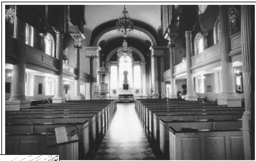
Interior of St. Paul's Chapel
