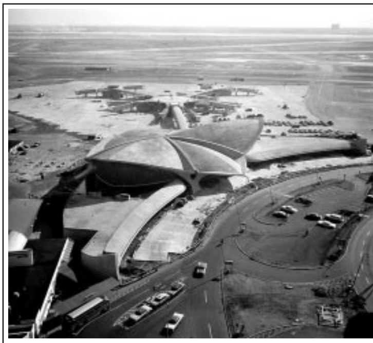
Aerial photograph of the TWA terminal under construction - from the files of the Port Authority of New York and New Jersey.
