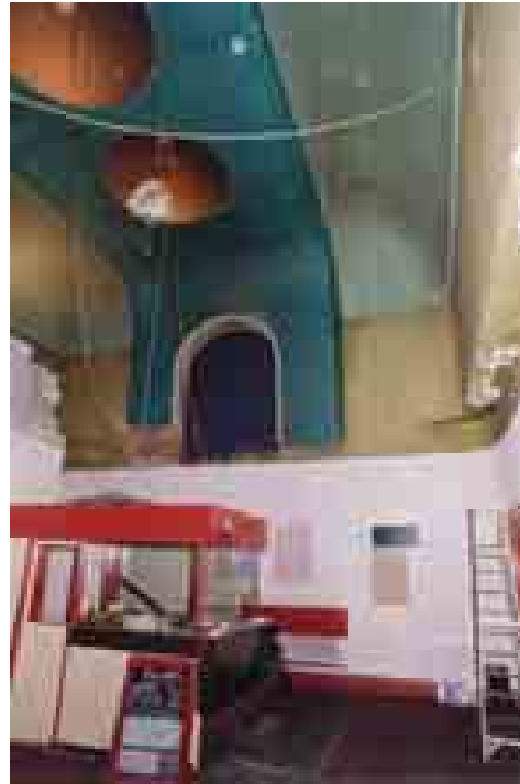
Fig. 5 Main Foyer 2001, view north-east
