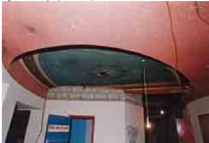
Fig. 11 Stalls foyer, view north-east showing later projection box
