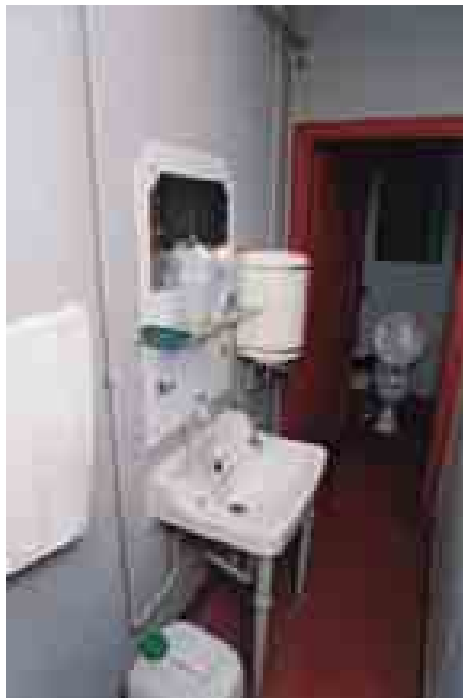
Fig. 12 Manager's office washroom
