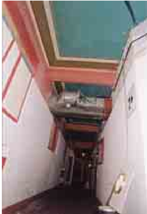
Fig. 10 Stalls foyer (50-57-27A) view south-west
