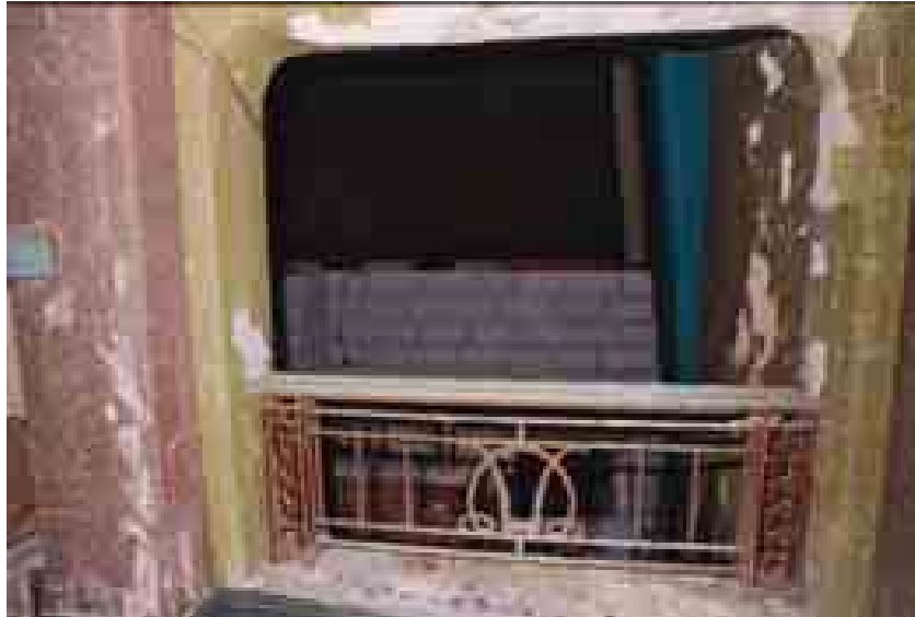
Fig. 8 Surviving arch, view south into main foyer
