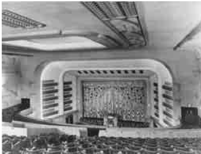
Fig. 23 Main auditorium in 1936 view NW
