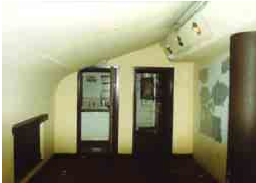
Fig. 16 Balcony foyer. Boxed-in NE alcove with two doors to ?kitchen
