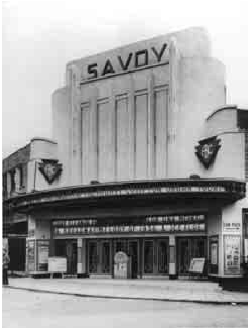
Fig. 2 The Savoy, Northampton in 1936. Main south-facing facade
