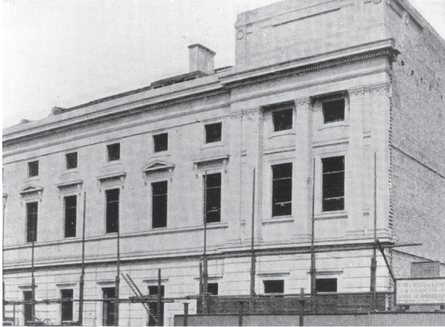
FIG. 10. The Bartlett Building near completion in the summer of 1914.
