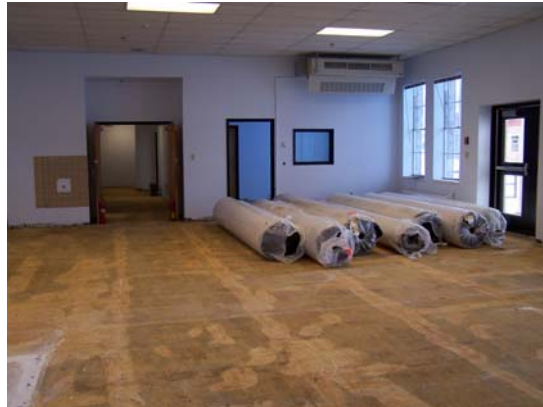
The building during renovations
