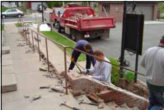
George Siegfried Construction rebuilt the handicapped ramp wall
