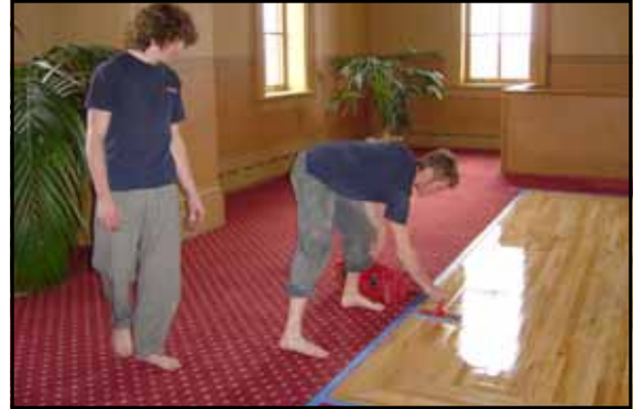
The dance floor and north lobby stairs and mezzanine were refinished
