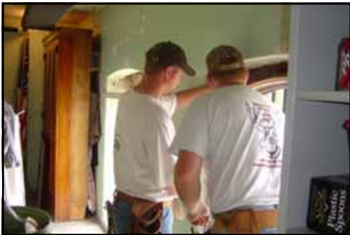
Parkos Construction installed new windows in jail
