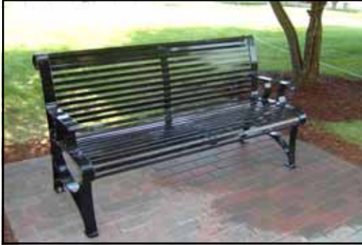
Three new benches and pavers were installed on the west side of the courthouse
