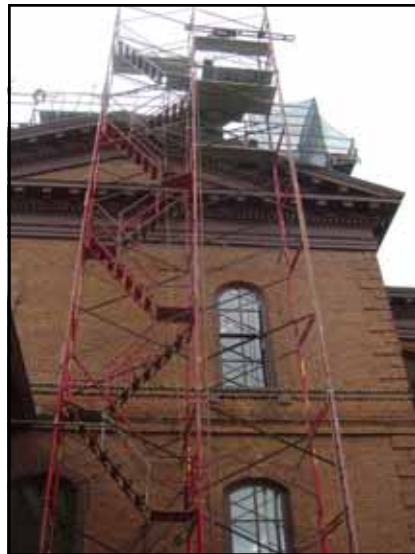
The final three chimneys were rebuilt during the summer
