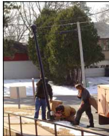
A light post was reinstalled after repairs
