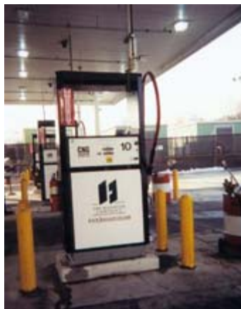
Figure 7. CNG Fueling Dispenser at WMATA
