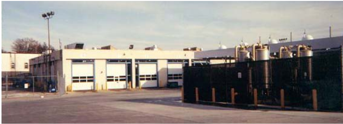
Figure 8. Maintenance Facility at Bladensburg
