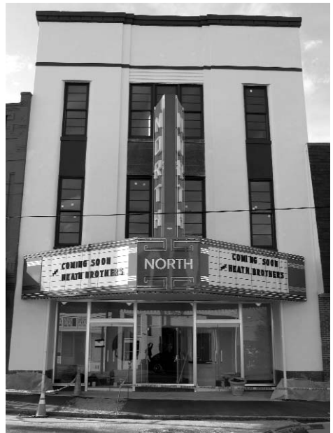
The North Theater after restoration of its marquee, windows, and façade to their 1947 configuration. The theater's historic interior features include decorative trim and light fixtures, terrazzo flooring, and lobby and balcony stairways with metal balustrade.
