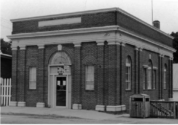
Bank of Louisa building (c. 1909) in Mineral Historic District
