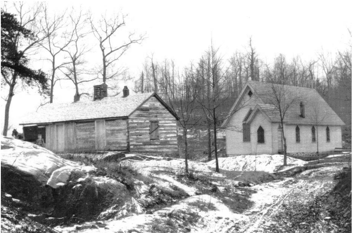
The Bear Mountain Indian Mission School (left) and St. Paul’s Mission Church (right), photographed in 1914, were part of an Episcopal mission established in 1908 to serve the Monacan community. Members of the community and a few white citizens constructed the church in 1908 and added a frame extension to an existing log schoolhouse that reportedly dates back to 1868. Today, the school building, which closed its doors as a school in 1964 with the advent of desegregation, is listed on the Virginia Landmarks Register and the National Register of Historic Places and serves as a museum. (Photo: Jackson Davis Papers, Special Collections, University of Virginia Library)
