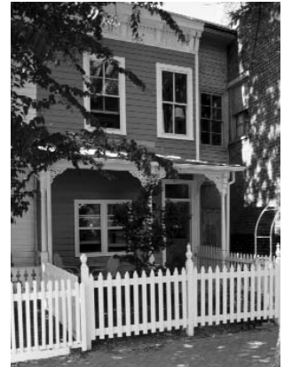
402 South Laurel Street
