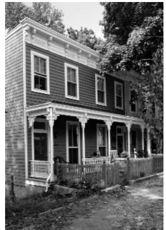
608 & 610 South Laurel Street
