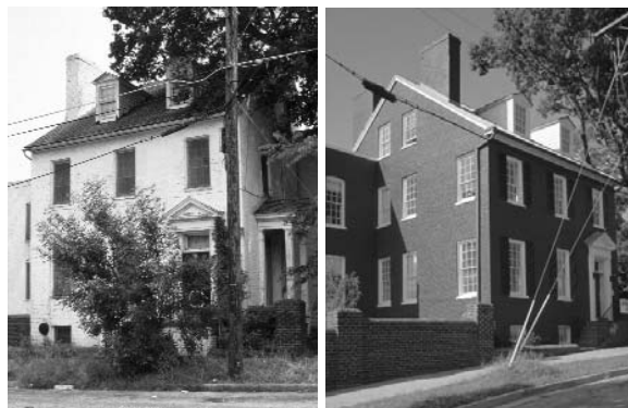
Parsons House, Oregon Hill, Richmond: In recent years the Parsons House had stood abandoned and in serious disrepair (left), until developer Robin Miller purchased the property from the state and undertook its rehabilitation (right). It is now one of the architectural highlights of the historic Oregon Hill neighborhood.
