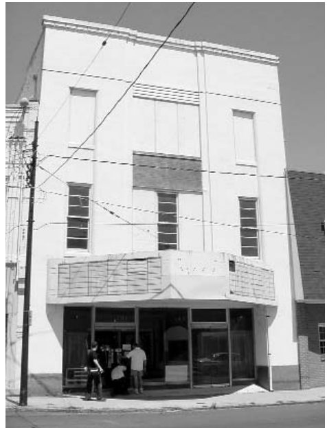
Danville's North Theater before restoration: The building was constructed circa 1900 and converted to a theater in 1947, with architectural modifications at the time that incorporated stylized Art Deco elements, the most prominent being the building's stucco façade.
