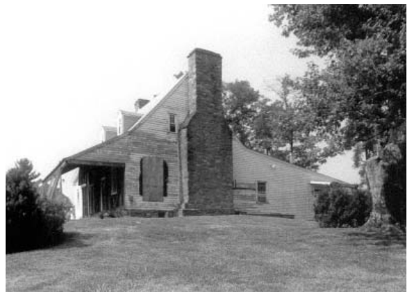
The former tavern-dwelling at Yew Hill during renovation
