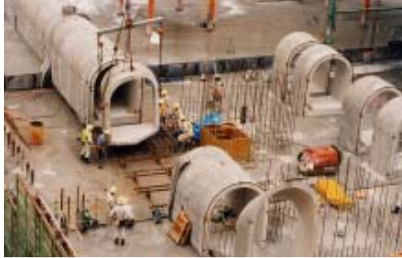
Fig.7 Example of Using Precast Gallery(Unazuki Dam)
