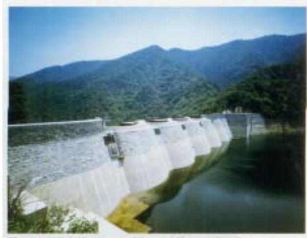
Fig.18 Upstream View of Honen-ike Dam After Treatment
