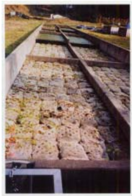
Fig.22 Phosphorus Absorption Materials(Terauchi Dam)
