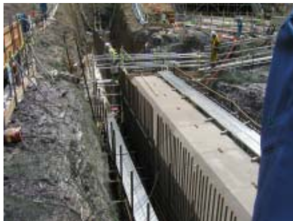
Fig.9 Example of Using Precast Gallery(Tokuyama Dam)
