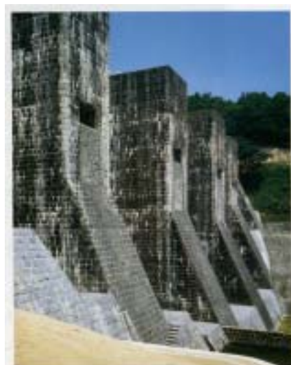
Fig.19 Downstream View of Honen-ike Dam after Treatment
