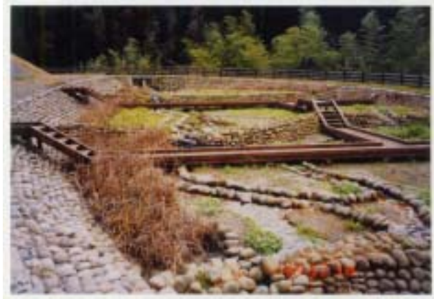
Fig.21 Cleansing Using Waterborne Plants(Terauchi Dam)
