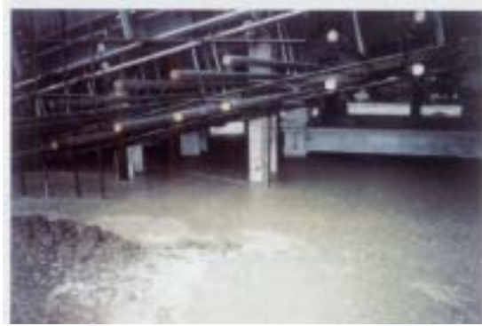
Fig.4 Placing of Self-compacting Concrete(Hinachi Dam)
