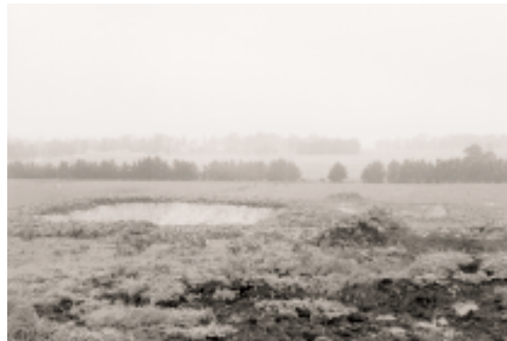
Photo: New aerobic pond under construction at Judson Park
