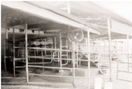
Photo: Newly completed dairy at Judson Park
