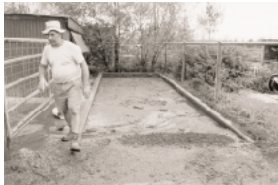
Photo: Valtin Campbell with the solids trap — part of the dairy effluent recycling system on Bickley Vale
