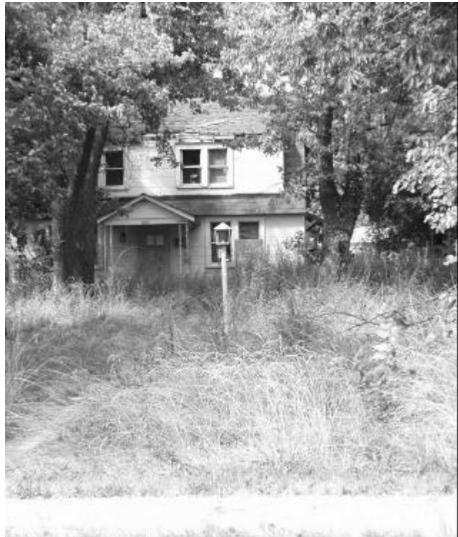
Example of high grass in a residential area.
