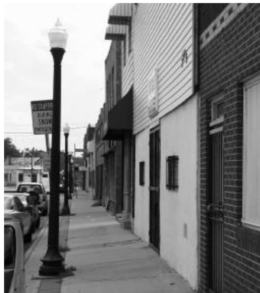
Existing commercial structures on Cleveland Avenue.
