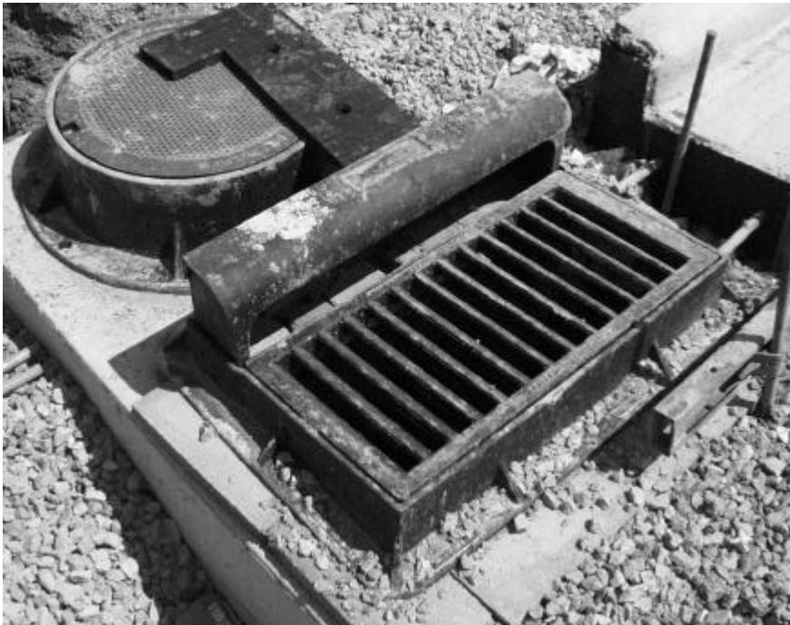
Sidewalk and curb being installed.
