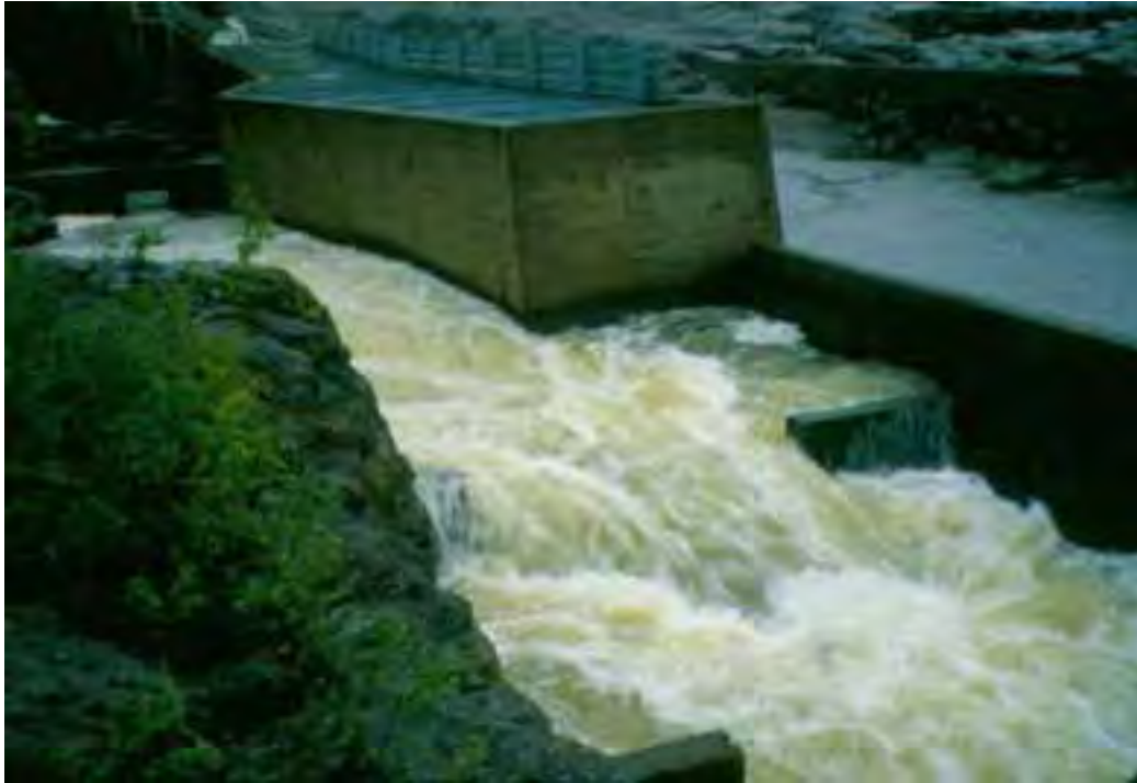
Figure 3. Norrfors Dam fish ladder entrance in upper left of photo and auxiliary water supplied to weirs downstream of the ladder entrance showing aerated, turbulent flow.
