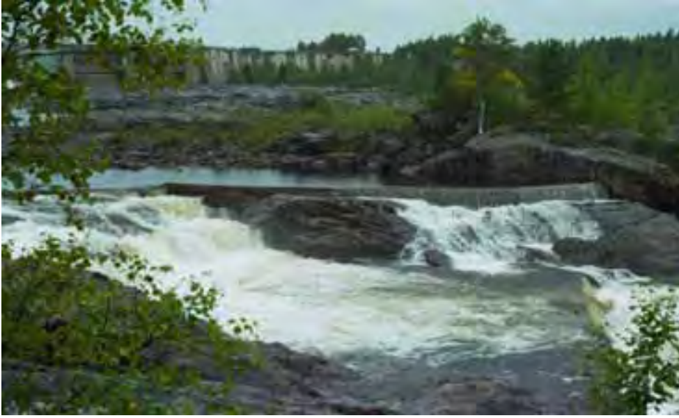
Figure 9. Laxhoppet area of natural falls and chutes has been modified to improve passage in the bypass reach under reduced flow conditions. Strategically placed weirs create 2 or 3 routes for fish passage.
