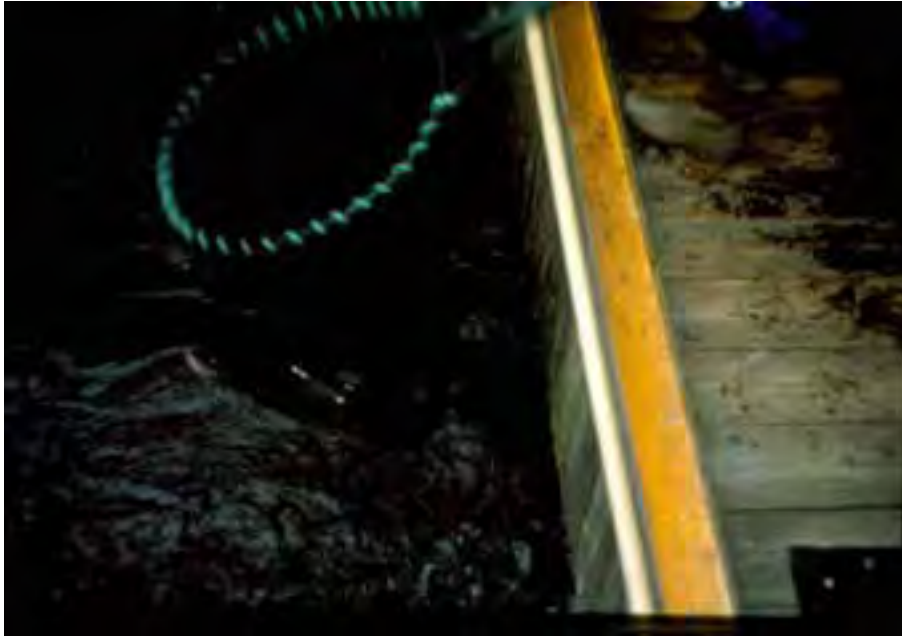
Figure 5. The adult collection facility is located in the top pool of the fish ladder. The pool is used to collect and hold fish, and the floor has a sloped rail that is raised to crowd adults for netting.
