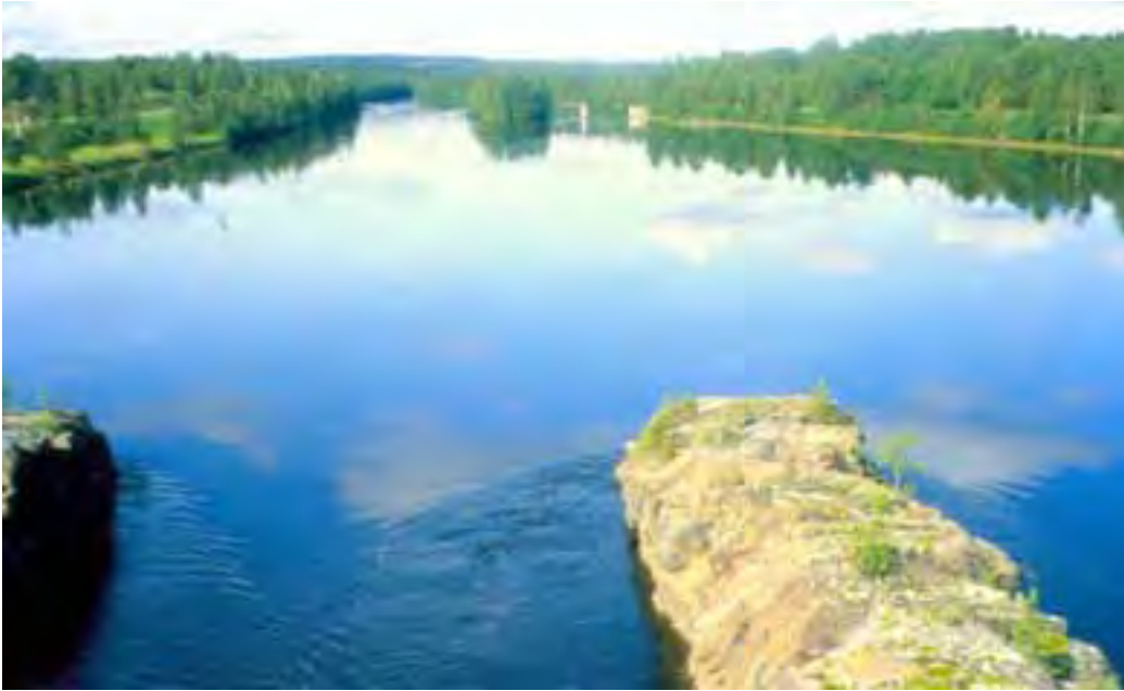
Figure 15. Stornorrfors Power Station intake channel where a juvenile salmon louver bypass system could potentially be installed. Flow between the rocks leads to each turbine.
