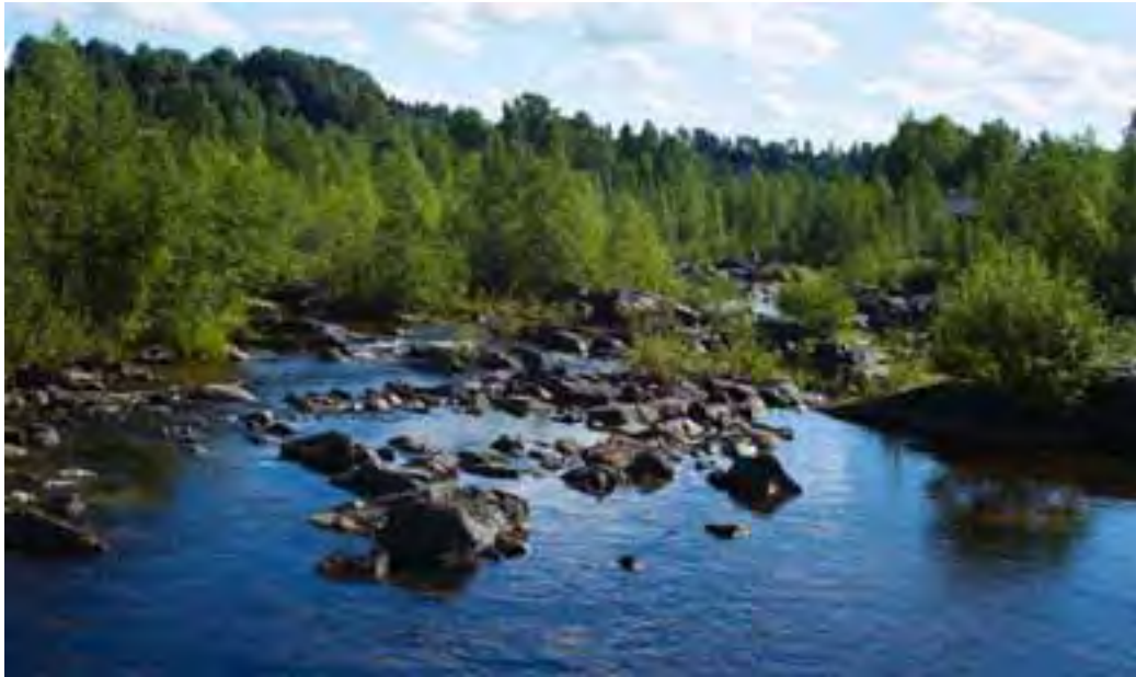
Figure 13. Approximately 20 m 3 /sec flow down the bypass channel provides a number of routes, chutes, and stepped jumps between rock formations, boulders, and potential areas of passage around the Baggböle Rapids near the old powerhouse.
