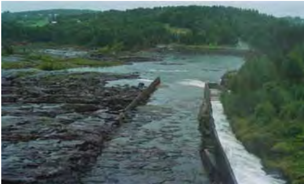
Figure 8. Spillway channel is comprised of rough, unfinished bedrock. The first energy-dissipating basin is downstream by the fish ladder entrance.
