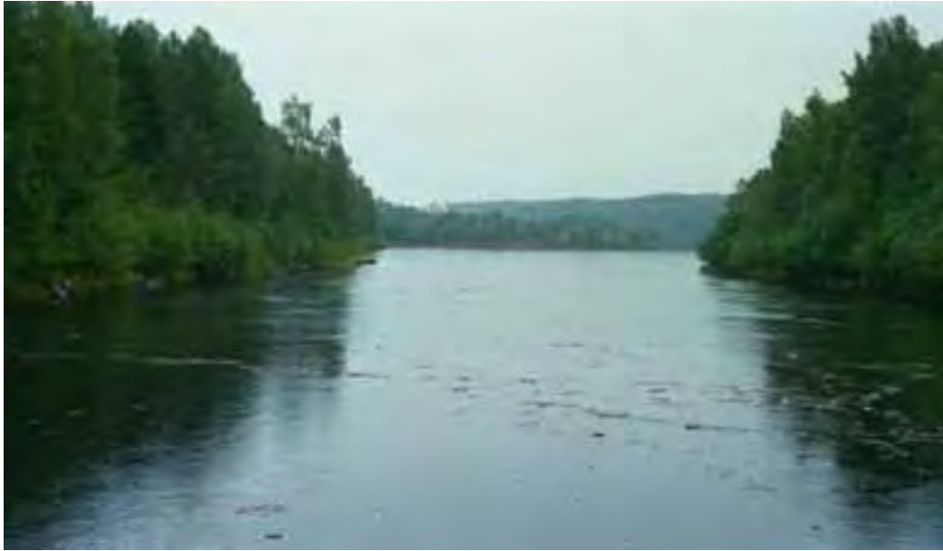
Figure 1. Stornorrfors Powerhouse tunnel tailrace, looking downstream (east).
