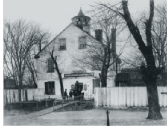
TUNNICLIFF'S TAVERN AT 9TH AND PENNSYLVANIA AVENUE, SE AND SHOWN IN THIS LATE 19TH-CENTURY PHOTOGRAPH OPENED IN 1795. WITHIN A FEW YEARS WILLIAM TUNNICLIFF MOVED HIS BUSINESS CLOSER TO THE CAPITOL. THE TAVERN LATER BECAME A HOTEL, PRIVATE HOME, AND BEER GARDEN BEFORE BEING DEMOLISHED IN 1936.
