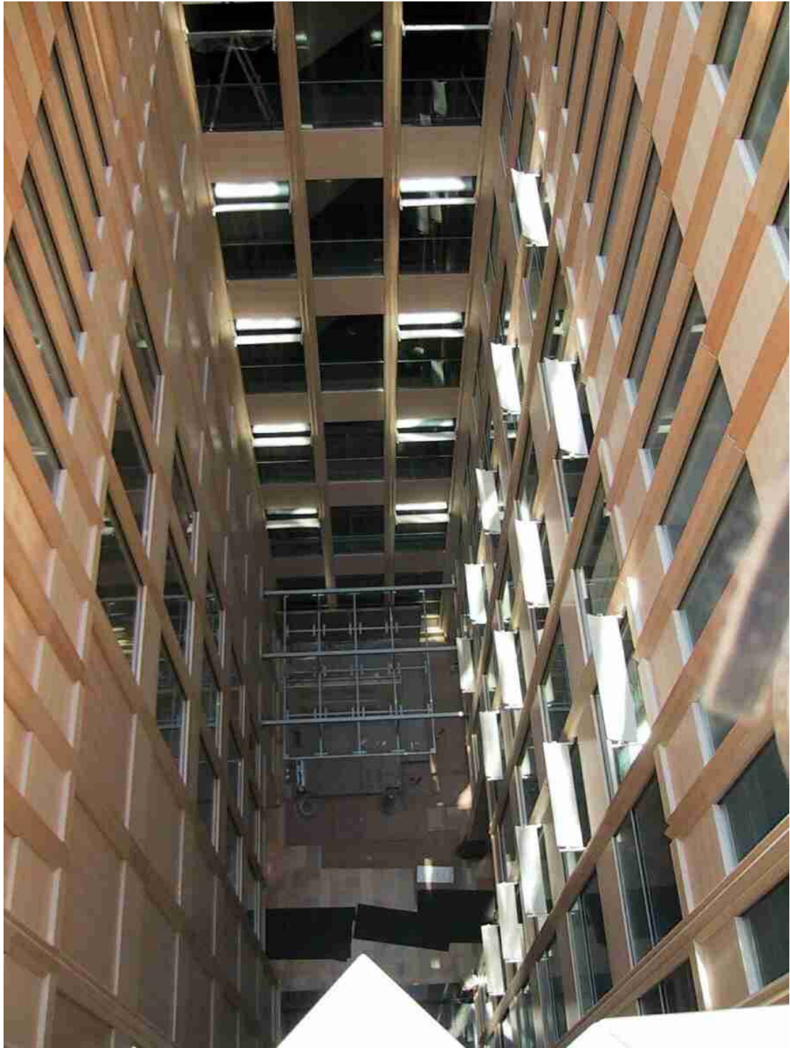
Figure 12: View down from the roof into the inner courtyard onto the second redirecting mirrors
