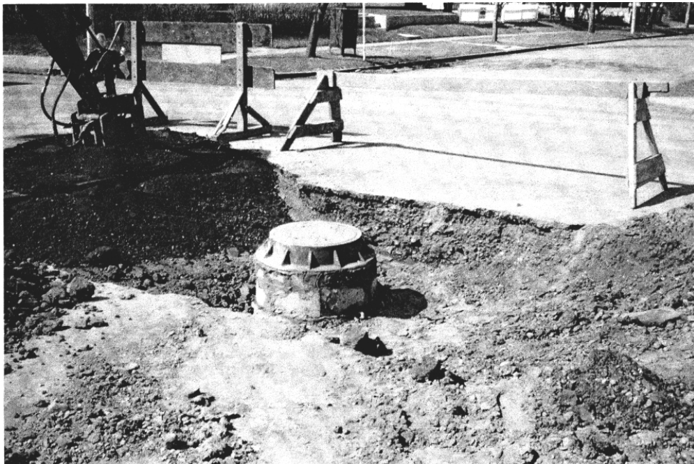
Upgrading of Water and Sewer Systems.
