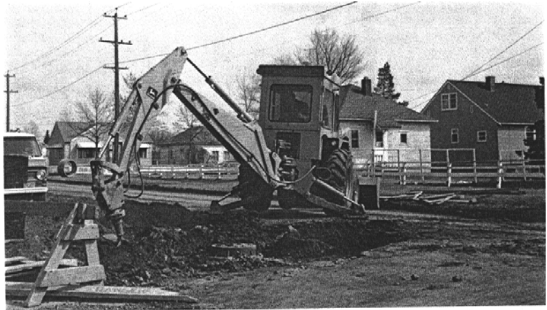
Sewer relief installation, 1978.
