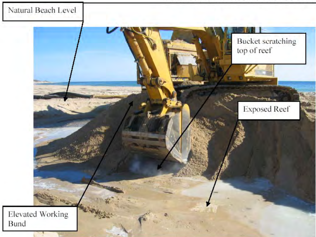
Figure 3 – Typical excavation at Dawesville; note exposed rock reef (JFA, 2005)
