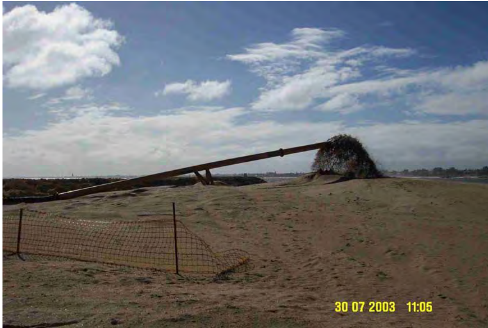
Figure 5 – Disposal of spoil at Mandurah by ‘rainbow’ discharge
