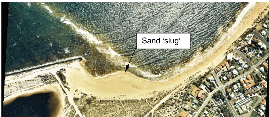
Figure 7 – Aerial Photograph: Mandurah, September 1996
