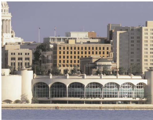
Madison's Monona Terrace Community and Convention Center is earning a "green building" certification with help from MGE.
