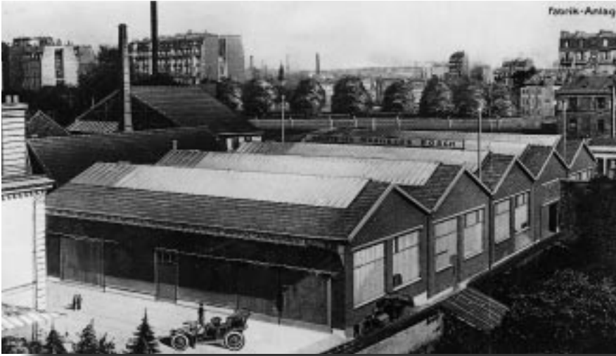
Bosch plant in Paris, 1905
