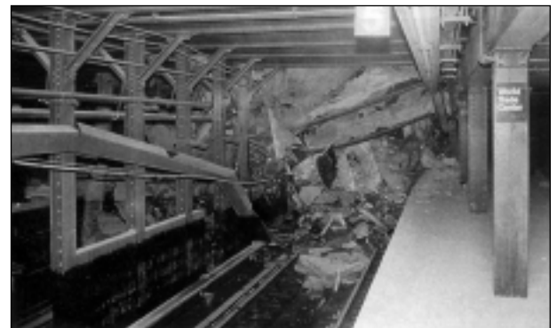
FIGURE 9 Damaged subway tunnel.
