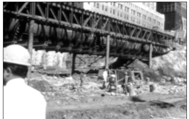
FIGURE 4 Original PATH tube suspension system.
