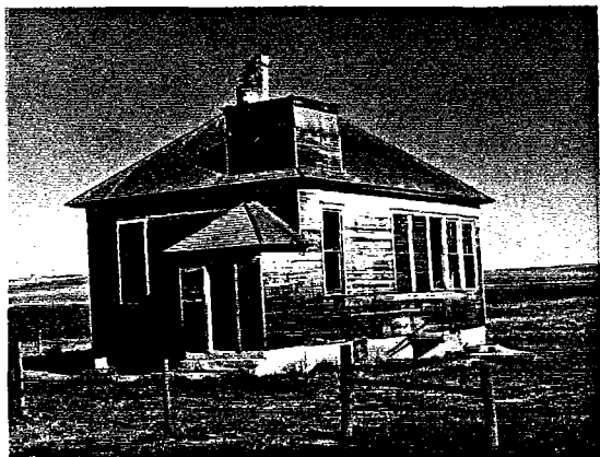
CD00-50: Abandoned School, ca. 1888. SW 1/4, SW 1/4, Sec. 15, T.30 N., R.1 W., Cedar County. Potentially eligible for NRHP listing based on association with recommended Multiple Property Nomination of hall-type school buildings in Cedar County.
