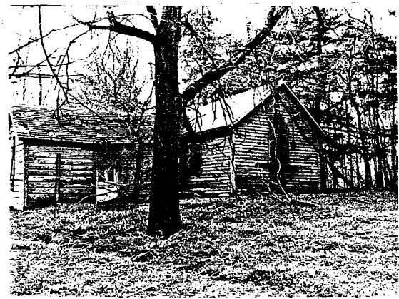
CD14-4: Abandoned House
