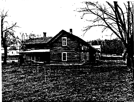
CD14-3: Abandoned House
