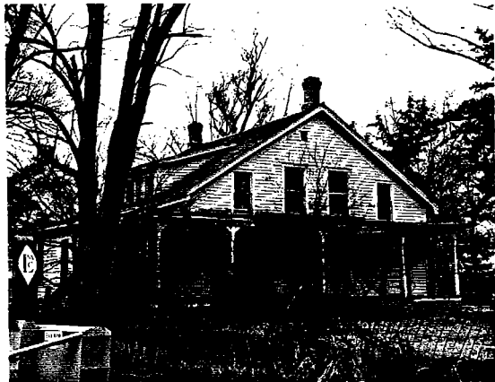
CD00-22: Abandoned House
