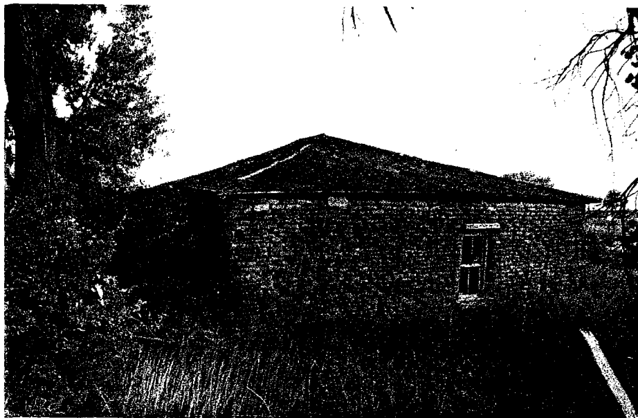
Fig. 5: Abandoned sod house rural Morrill County (MO00-099).
