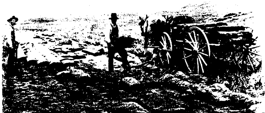
Fig. 6: Loading sod for building a sod house near Dismal River in Thomas County. (Photo: Nebraska State Historical Society).
