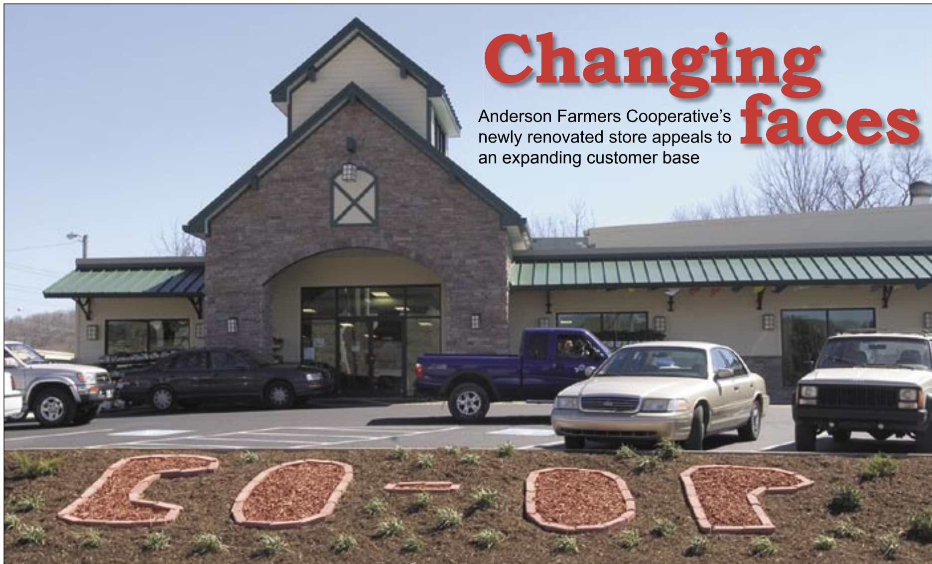
Located on a bustling street in downtown Clinton, Anderson Farmers Cooperative's newly renovated store attracts a wide range of customers. Manager Anthony Hastings says the Co-op's board of directors wanted to build a store that would be strikingly noticeable while maintaining a "hometown" appeal.
