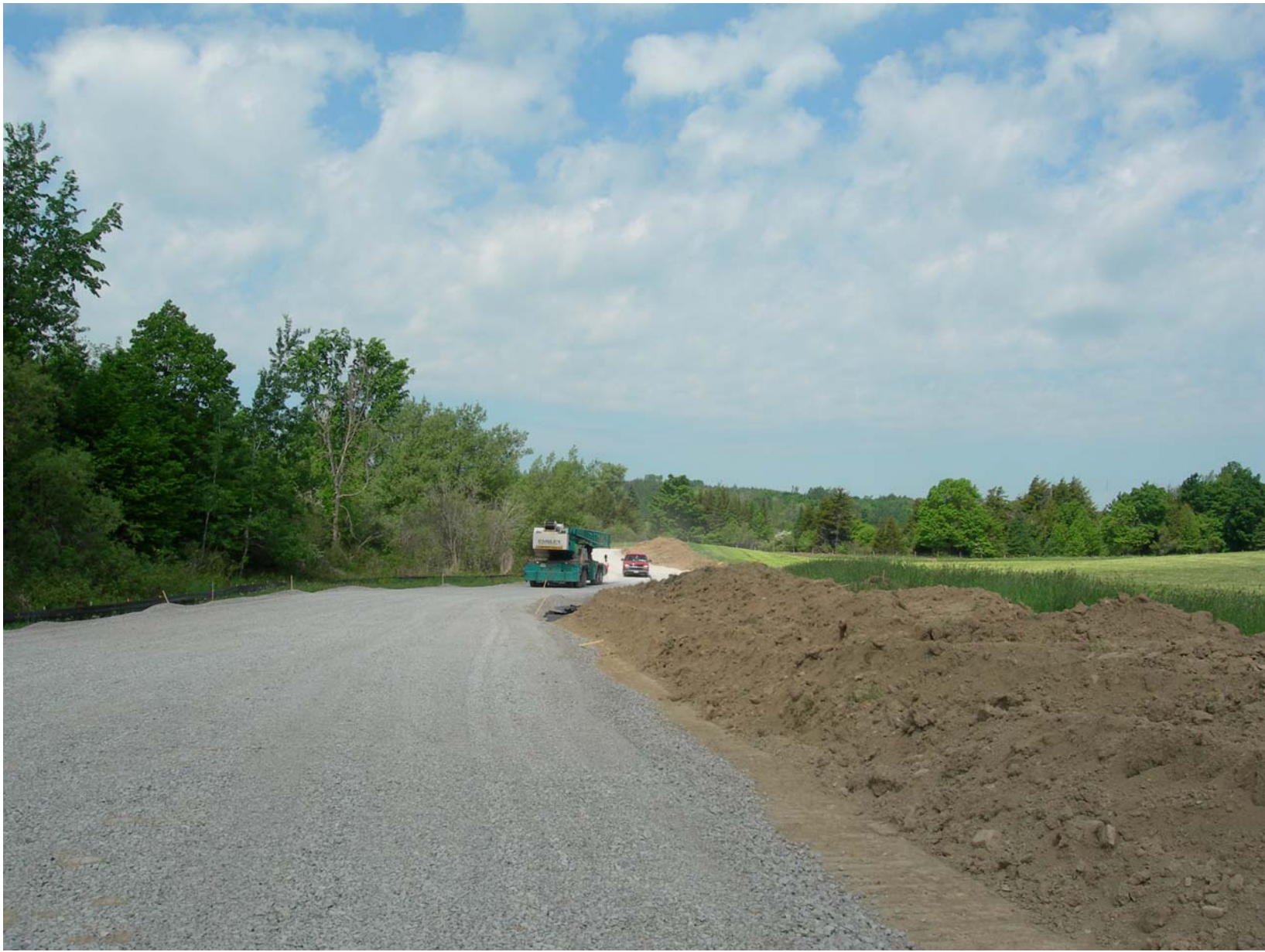
Access road located along field edge to minimize disturbance to field and cropping pattern.
