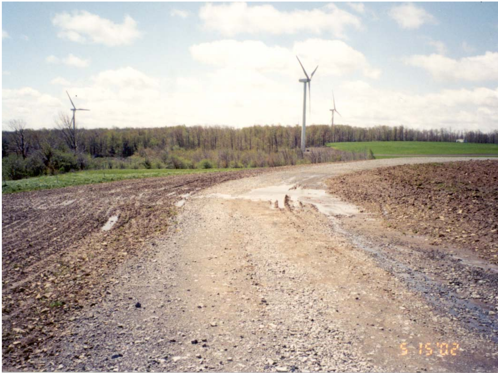
This slide shows the soil saturation problem caused in the field on the left side of the access road. These types of drainage problems must be corrected to prevent damage to the fields.
