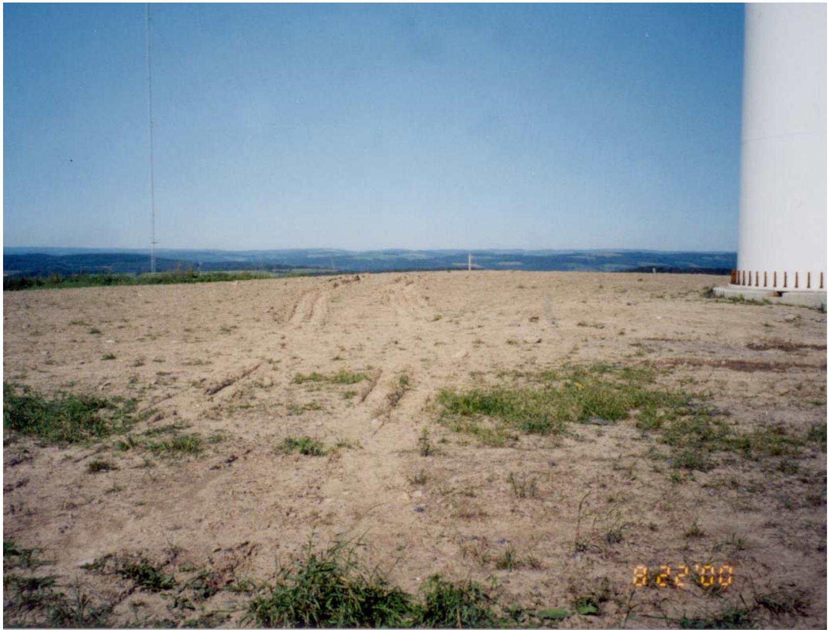
Seeding failed at the tower site because of lack of topsoil material on the surface. This photo was taken one year after the area was restored and seeded. Imported topsoil was required to establish a seeding.
