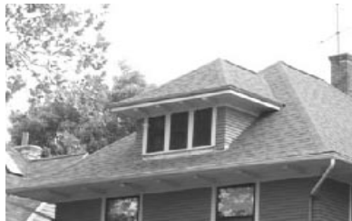
Hip roof and dormer
