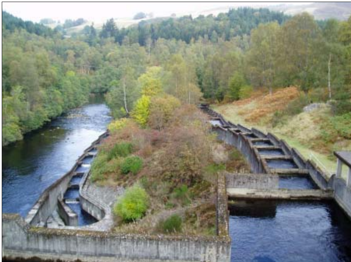
Plate 2. The fish ladder at Clunie dam on the River Tummel (Tay catchment). Reproduced courtesy of Dan Eatherley.
