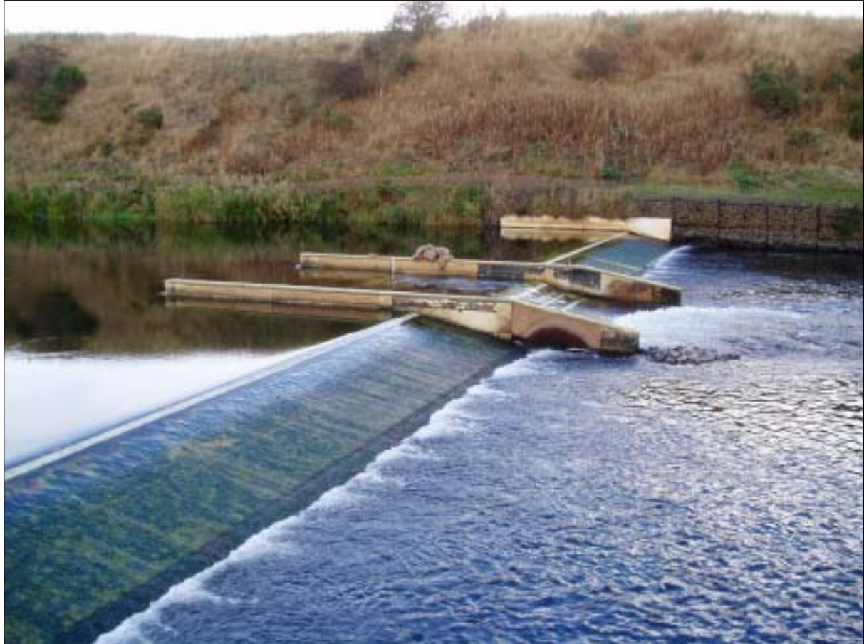
Plate 1. The 'Crump'-type weir with embedded counting electrodes at Logie on the River North Esk (North Esk catchment). Reproduced courtesy of Dan Eatherley.
