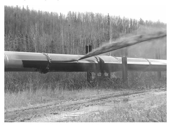
**Bullet Hole Spill:** After a drunken hunter shot the Trans-Alaska Pipeline north of Fairbanks in October 2001, crude oil gushed out at 100 gallons per minute for 36 hours until 285,000 gallons had pooled in the boreal forest and Alyeska Pipeline Service Co. plugged the hole. 12
