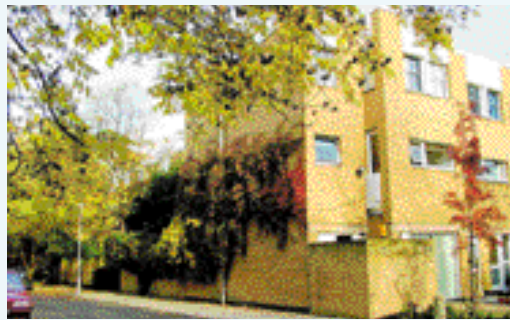
New planting has been introduced to soften building elements
