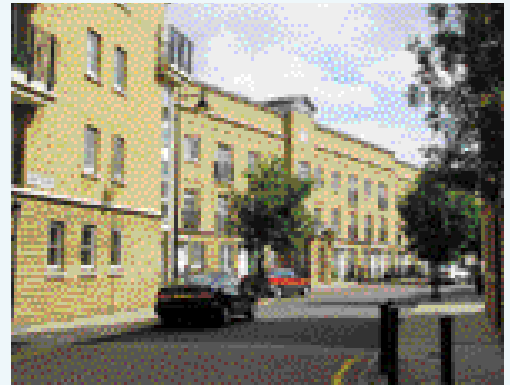
Here orientating the fronts of dwellings away from a dominating railway line is an important structuring element in the design. Isledon Village, Islington
