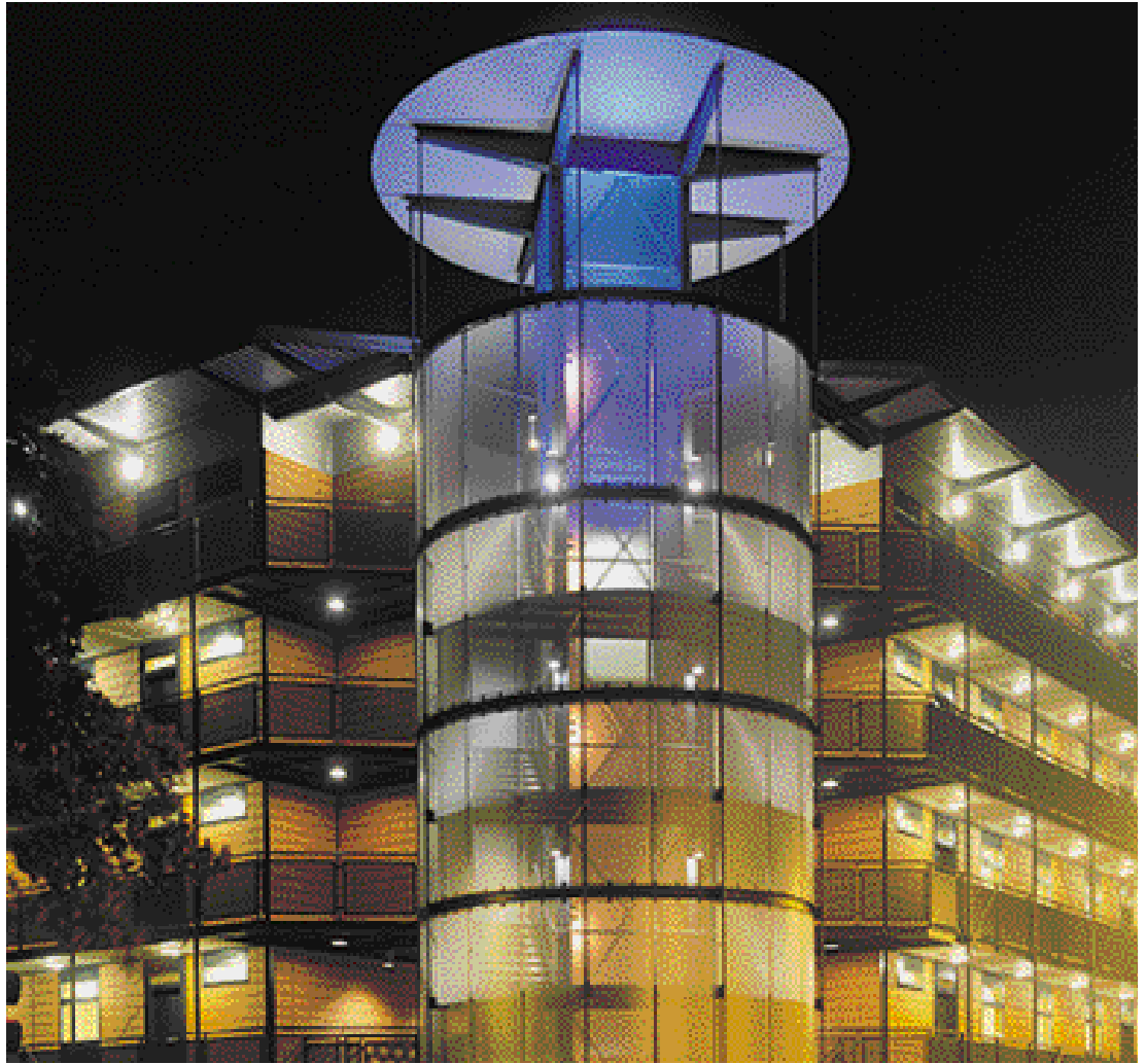
Design thinking, building technology and residents' aspirations are continually evolving. Murray Grove, Hackney
