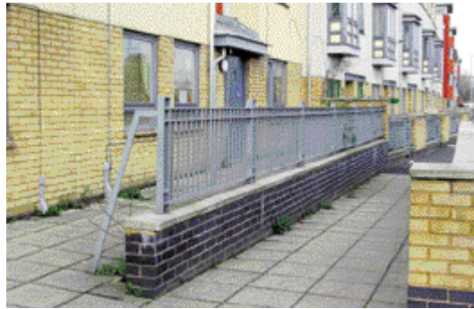
This wheelchair ramp has blurred the distinction between public and private space with the unintended consequence of providing a place for children to cycle and skateboard, causing nuisance to residents. Rolls Crescent, Hulme
