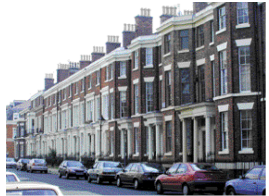
Certain historic housing forms have proved very adaptable to changing requirements. Here, large town houses built for wealthy merchants have been converted to apartments and offices. Canning Street, Liverpool
