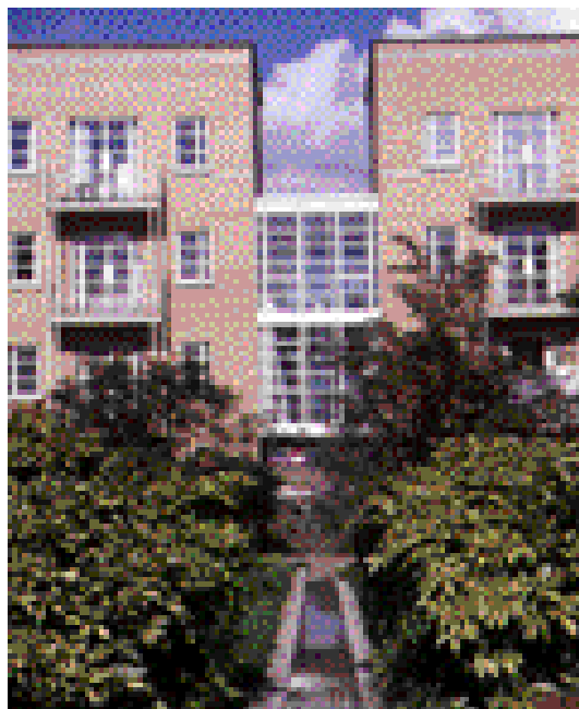
Denser urban apartment blocks require careful consideration to ensure good solar penetration to the interior of the block. Here a break in the building block at the third storey allows good sunlight penetration to an attractive communal space. Narrow Street, Tower Hamlets, London.
