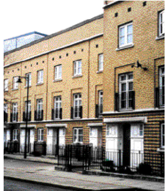
Smaller kitchen windows balance the need for surveillance with privacy. Isledon Road, Islington
