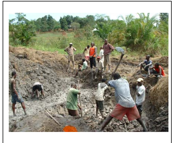
Students at Masooli Secondary School making bricks for their YEP! Enterprise.
