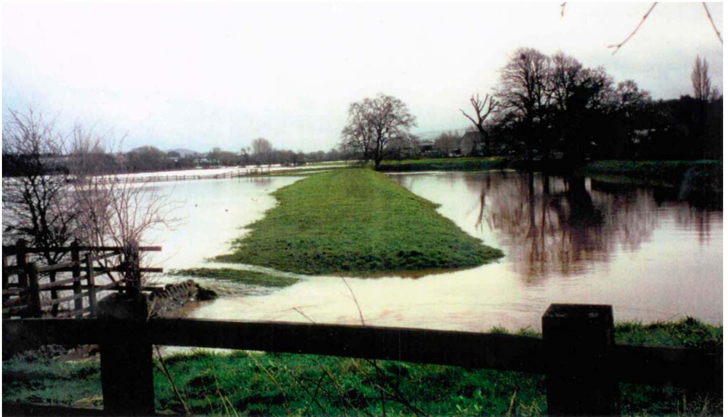
Floodwater from the River Yeo spills over on to fields upstream of the A370 road bridge at Congresbury
