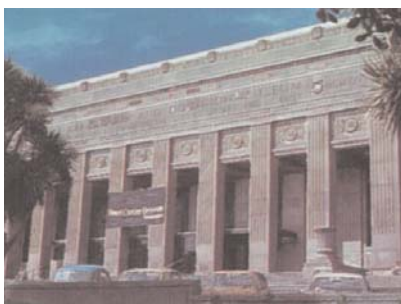
The old Dominion Museum building, Wellington
