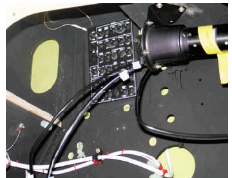
Circuit breaker panel and power distribution panel installation.
