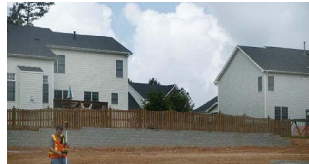
Figure 6 Poor Example of Wall Cladding Variety
