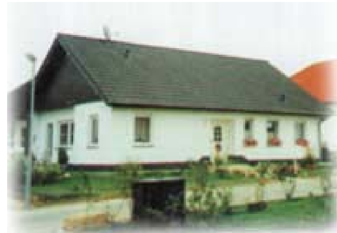
Figure 15 Example of Unacceptable Large Roof Areas
