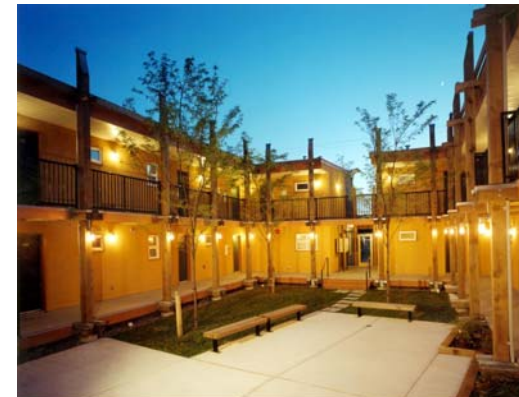
Figure 26 Example Site & Building Lighting
