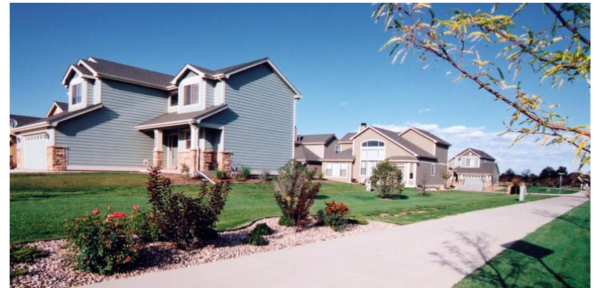
Figure 12 Example of blank walls without Fenestration
