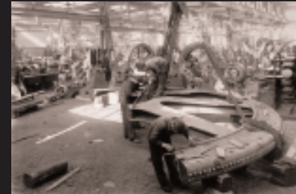
Generatormontage in Baden, 1895
