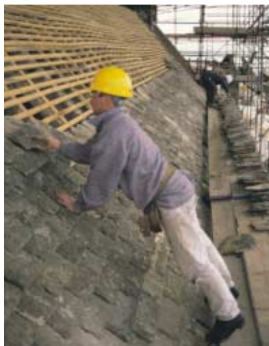
Trainee laying Forest marble stone slates
