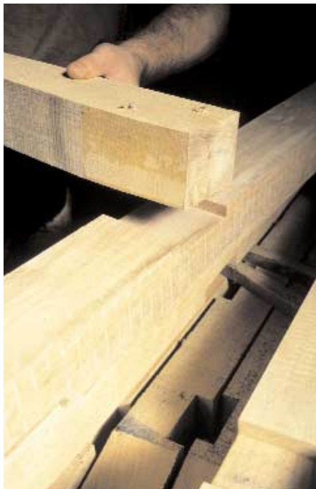
Oak frame prepared off site for construction
