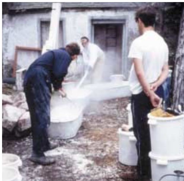
Trainees mixing plaster
