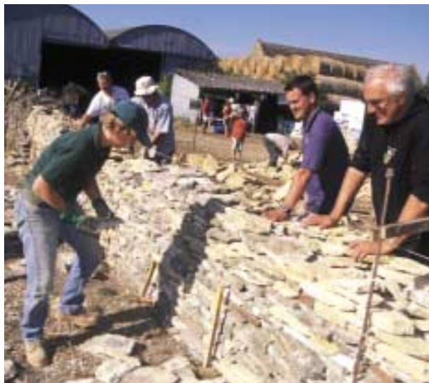
Dry-stone walling competition, Cotswolds AONB
