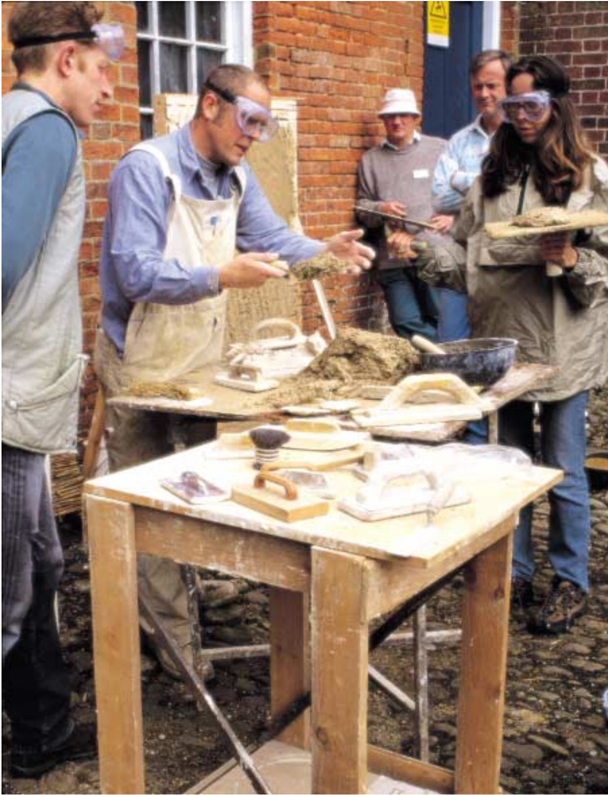
Demonstrating lime plasterwork
