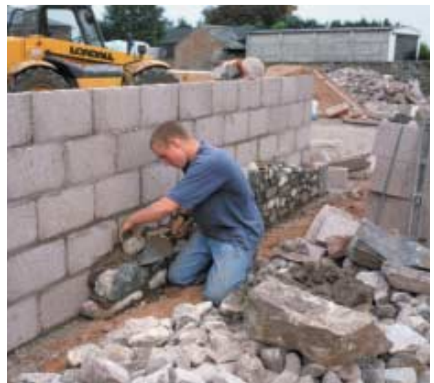
Coble facing wall to conform to District Council rules, Solway Coast
