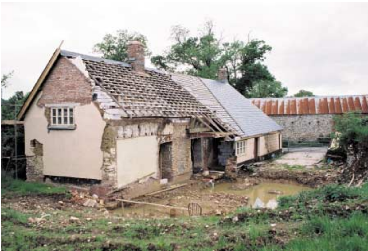
Major repair and extension to existing cottage
