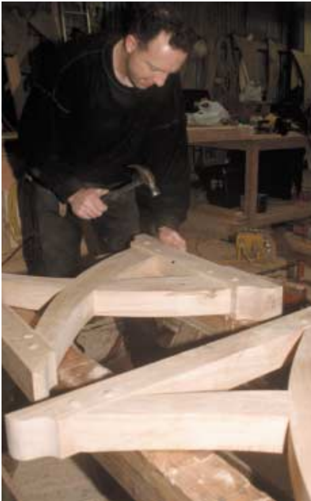
Constructing an oak frame, Holmsley
