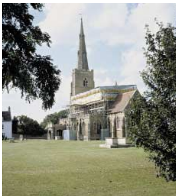
Renovation of St. Wendreda's, March, The Fens
