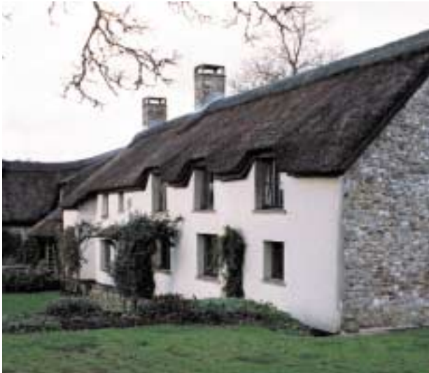
Barn Farm renovation, Luppitt, Blackdown Hills
