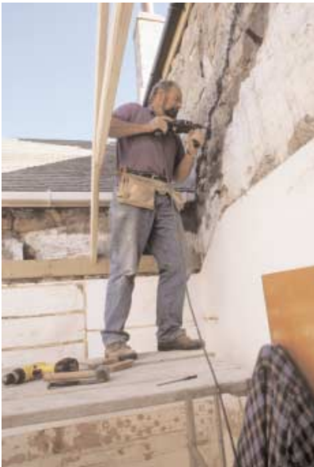
Renovation, Hugh Town, St Mary's, Isles of Scilly
