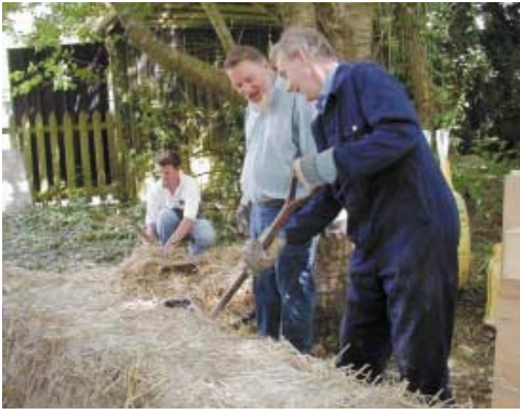
Cob-walling demonstration
