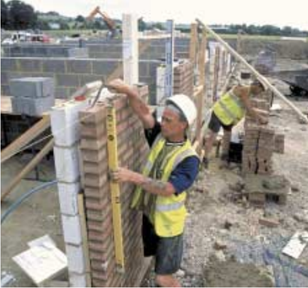
Building affordable homes, Kent
