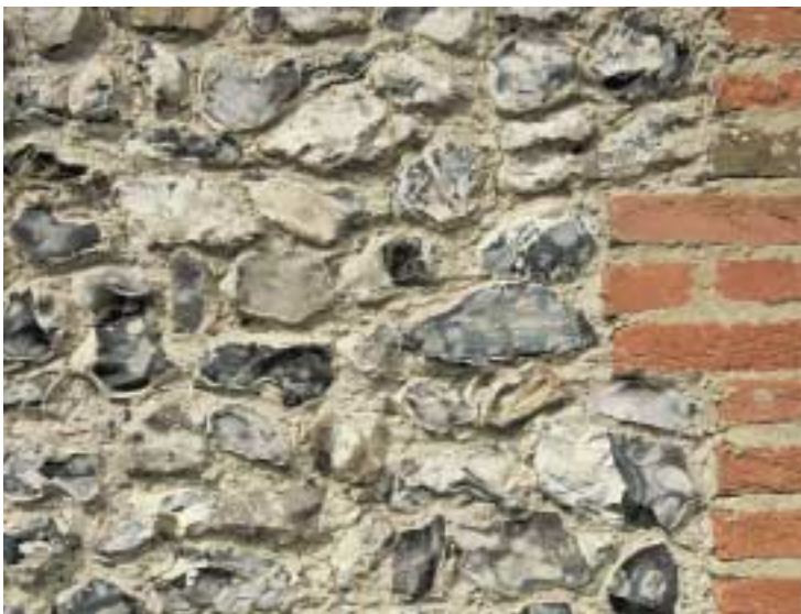
Flint and brick walling, Singleton
