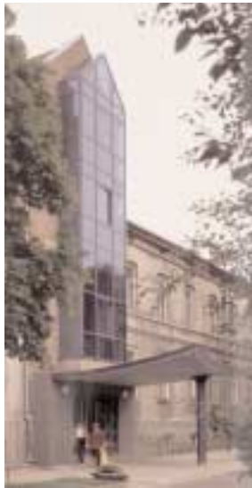
Entrance of the Faculty of Environmental Engineering
