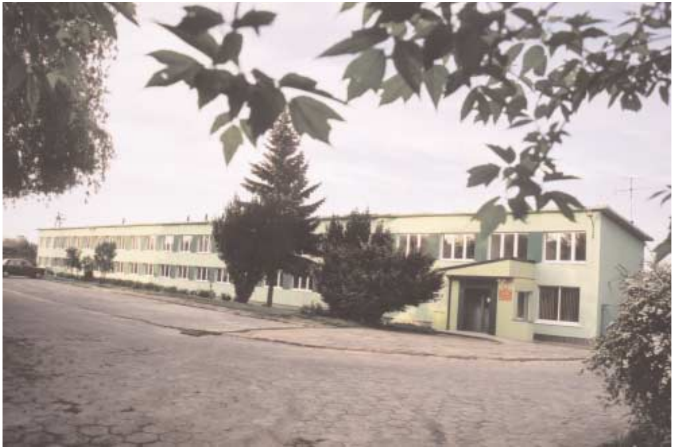
Building of the Institute of Environmental Protection and Engineering
