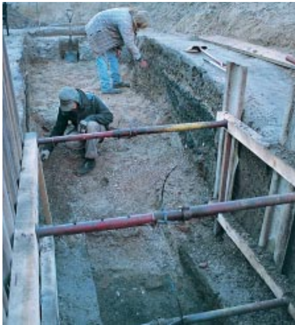
Landguard Fort: ditch excavation
