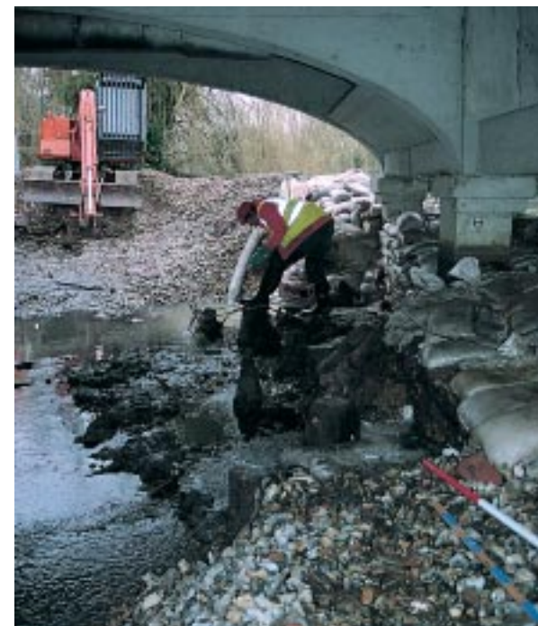
Ballingdon Bridge: Timber piles of an earlier bridge
