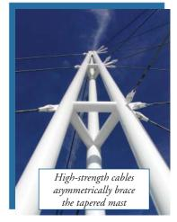
signed to minimize water infiltration and corrosion. The cable-stayed solution, along with a creative cable erection sequence that reduced the number of required shoring towers, reduced both construction time and cost of the overall project.
