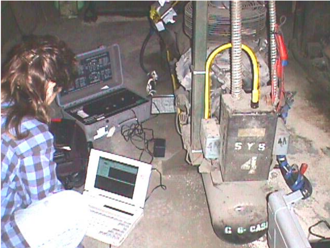
DWP technician downloads kW data monitored and logged by power recorder into laptop computer
